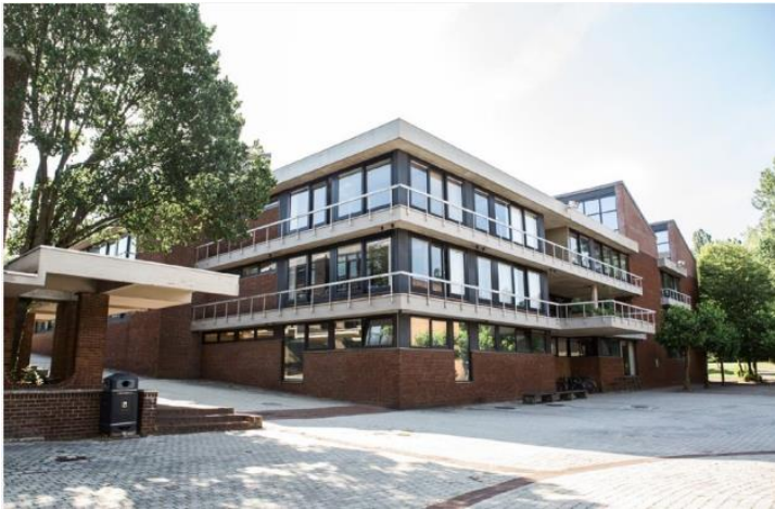
Case Study 1: The Vinci Building. Source: Baldwin et al., 2023
